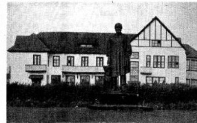
Building containing Pavlov's flat and the Laboratory of Academician Airapet'yan.
